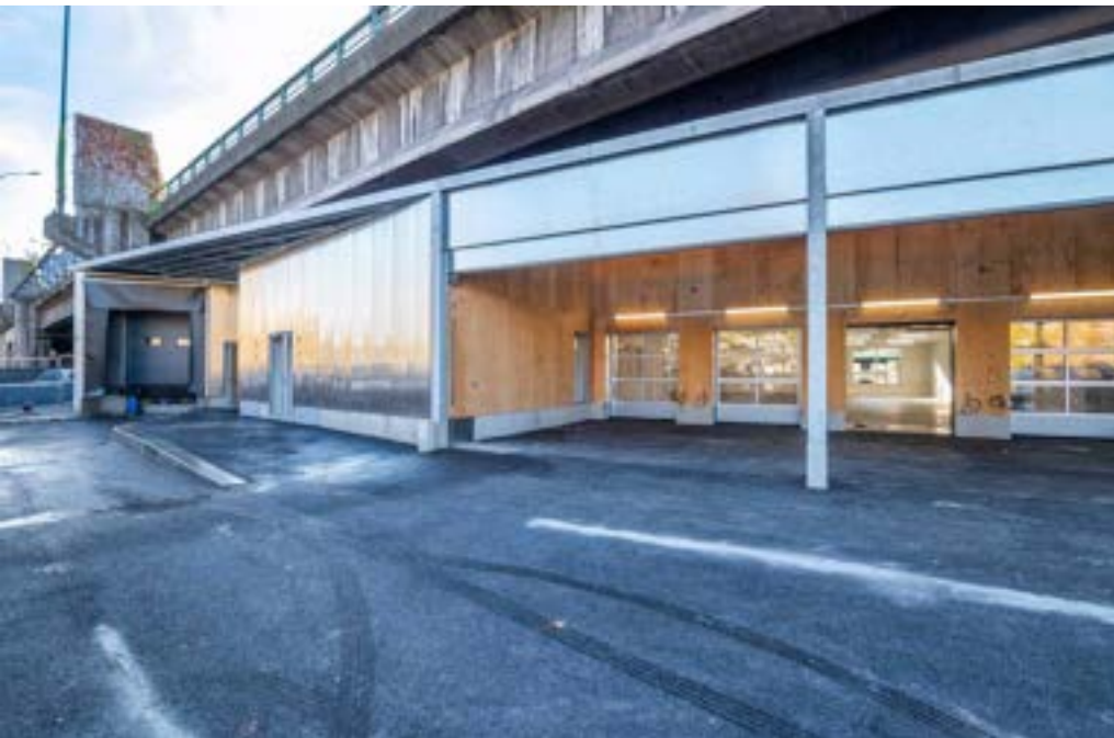
Microhub in Porte de Pantin, Paris, France / Source: Sogaris ©ThomasGarcia
