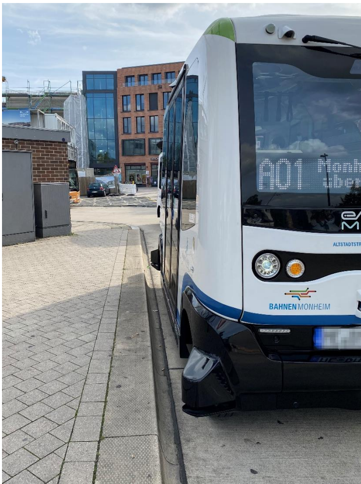
Figure 3: Bus stop no tactile ground markings
