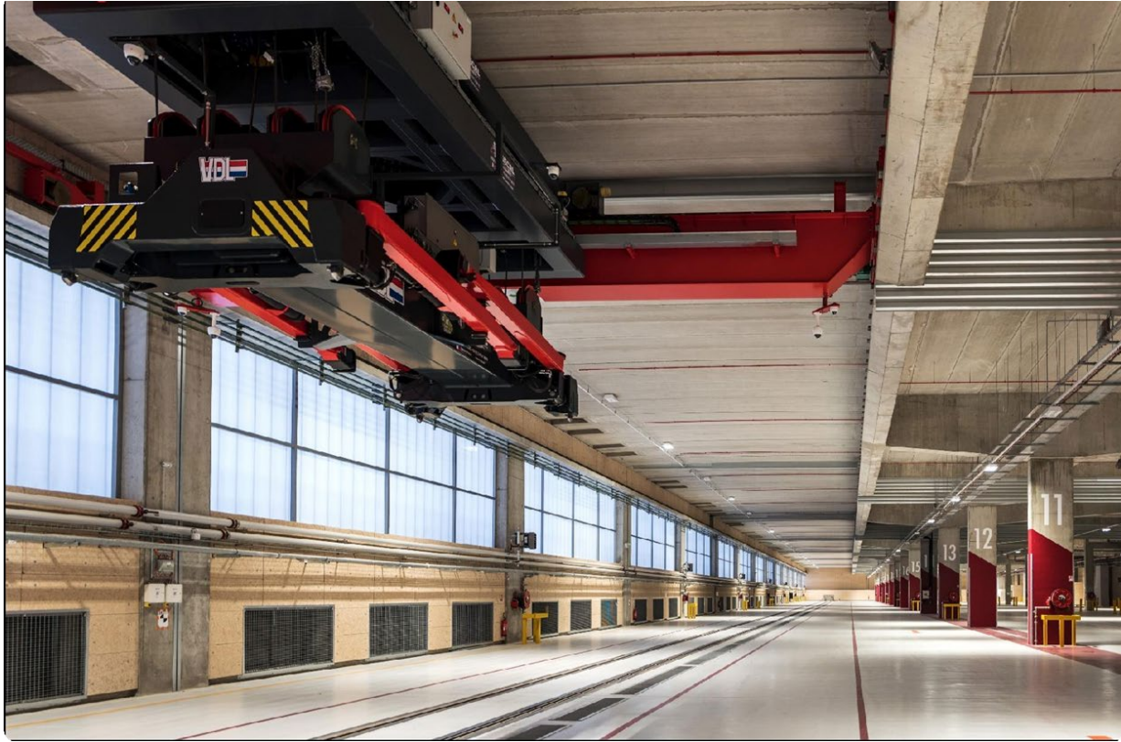
Figure 6. Logistics Hotel Chapelle International: Indoor rail terminal and cross docking
