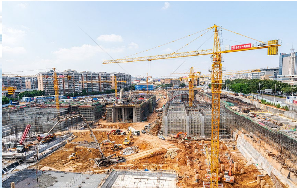
Traditional construction site.
