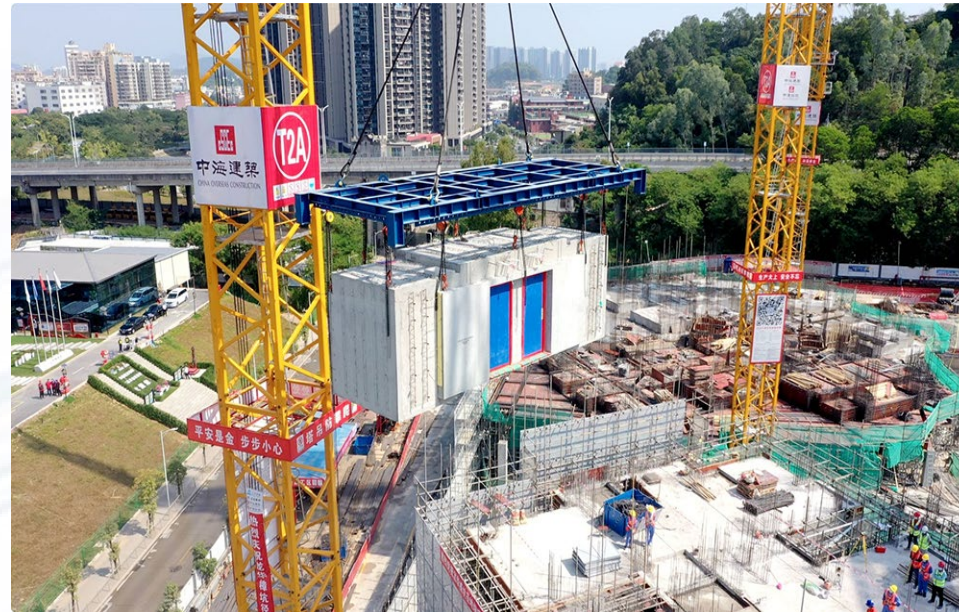
MiC construction site.
